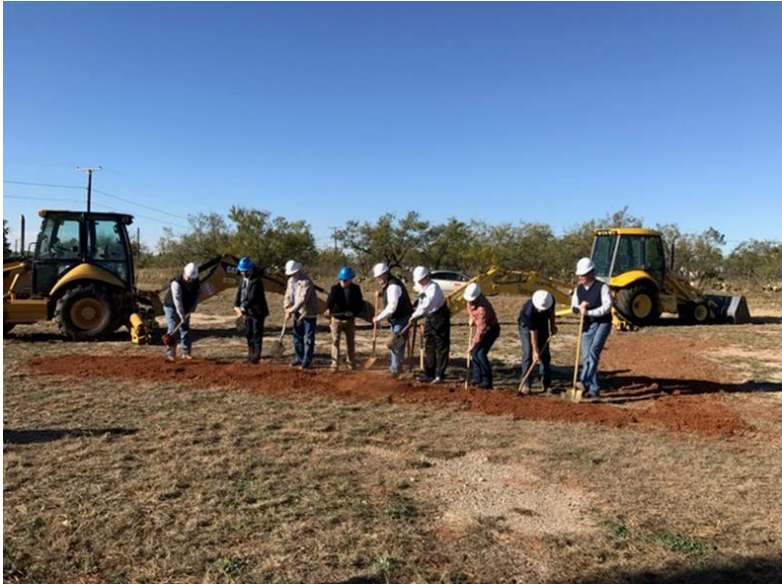
December 2016 Ground breaking
